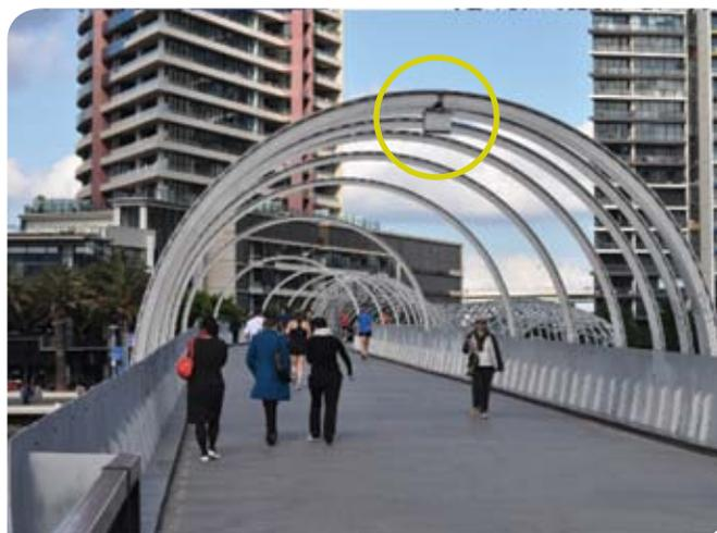
A passive infrared (overhead) pedestrian sensor at Victoria Point, 768 Bourke Road, Docklands and a laser sheet (overhead) pedestrian sensor at Webb Bridge, Docklands
